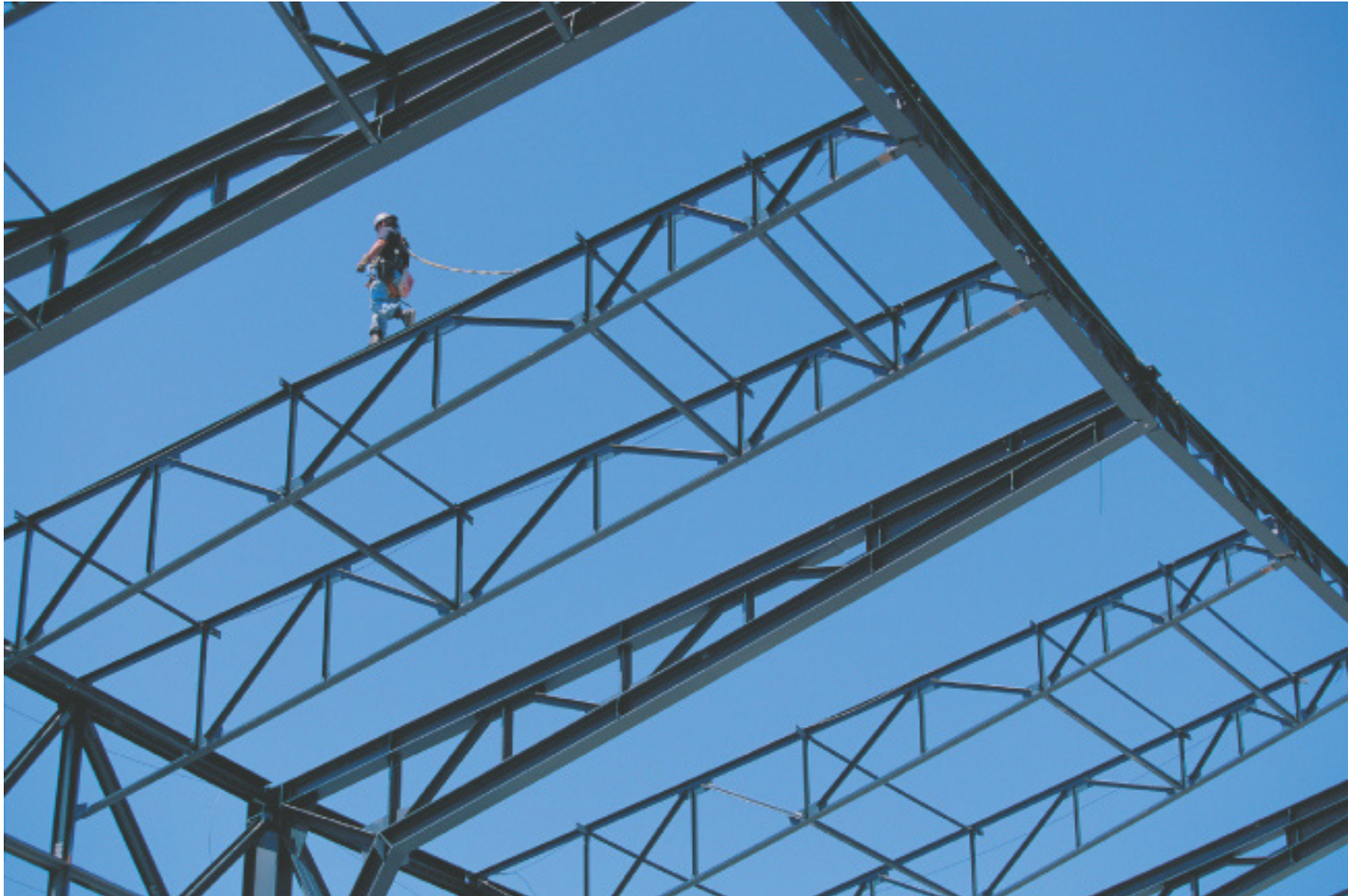
Roof trusses – Safeco Field in Seattle
