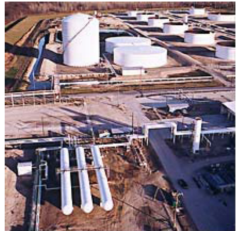
Cylindrical Pressure Vessels
