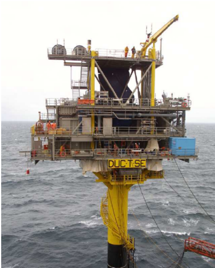
Tyra South – STAR platform
