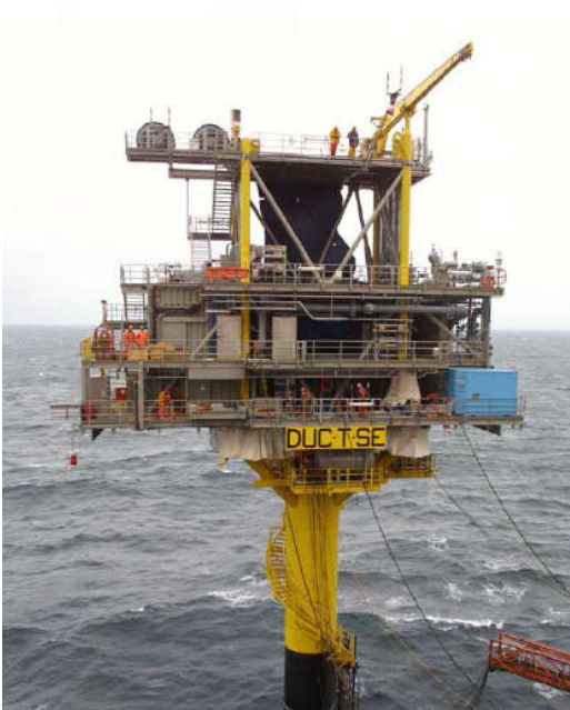
Tyra South – STAR platform
